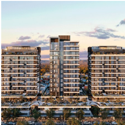
88 O'Connell Project Delivery
